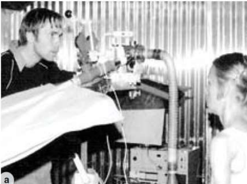
FIGURE 0.2 (a) Early measurements of metabolic responses to exercise required the collection of expired air in a sealed bag known as a Douglas bag. (b) A sample of that gas then was measured for oxygen and carbon dioxide using a chemical gas analyzer, as illustrated by this photo of Nobel laureate August Krogh.
