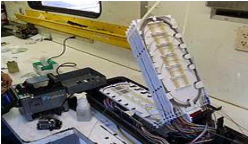
Underground fiber splice tray
