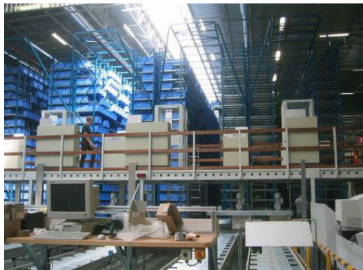
An automatic storage warehouse for small parts. Warehouses today are becoming increasingly automated – where robots do the work that humans used to.
