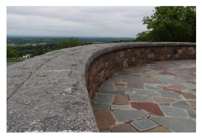
For constructing a flagstone floor, the same method is applied as in case of tile floor. The slabs are soaked well in water at least one hour before laying. They should be evenly and firmly bedded in mortar. The thickness of joints should not exceed 4mm and they should be struck off with a trowel while laying.
