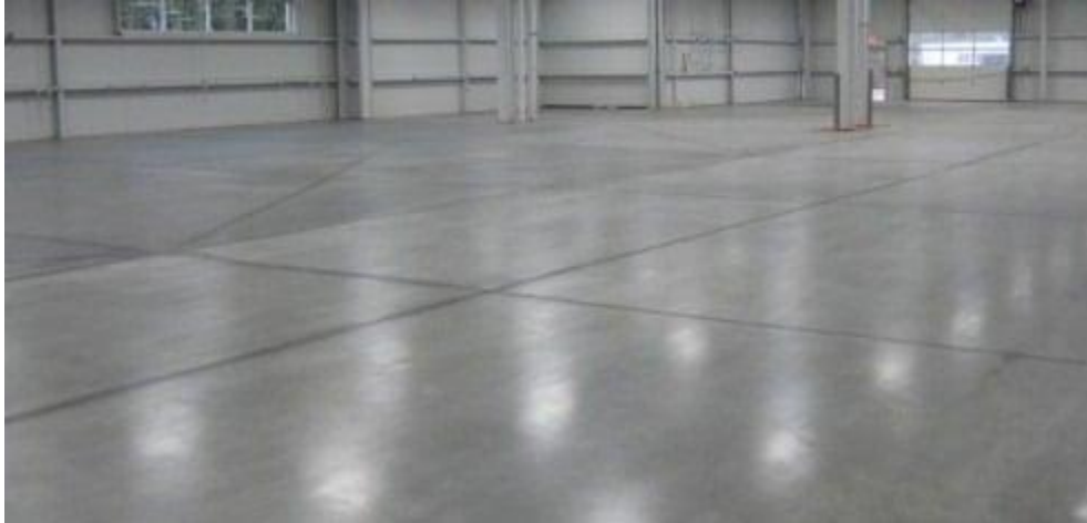
Fig: Cement Concrete Flooring
